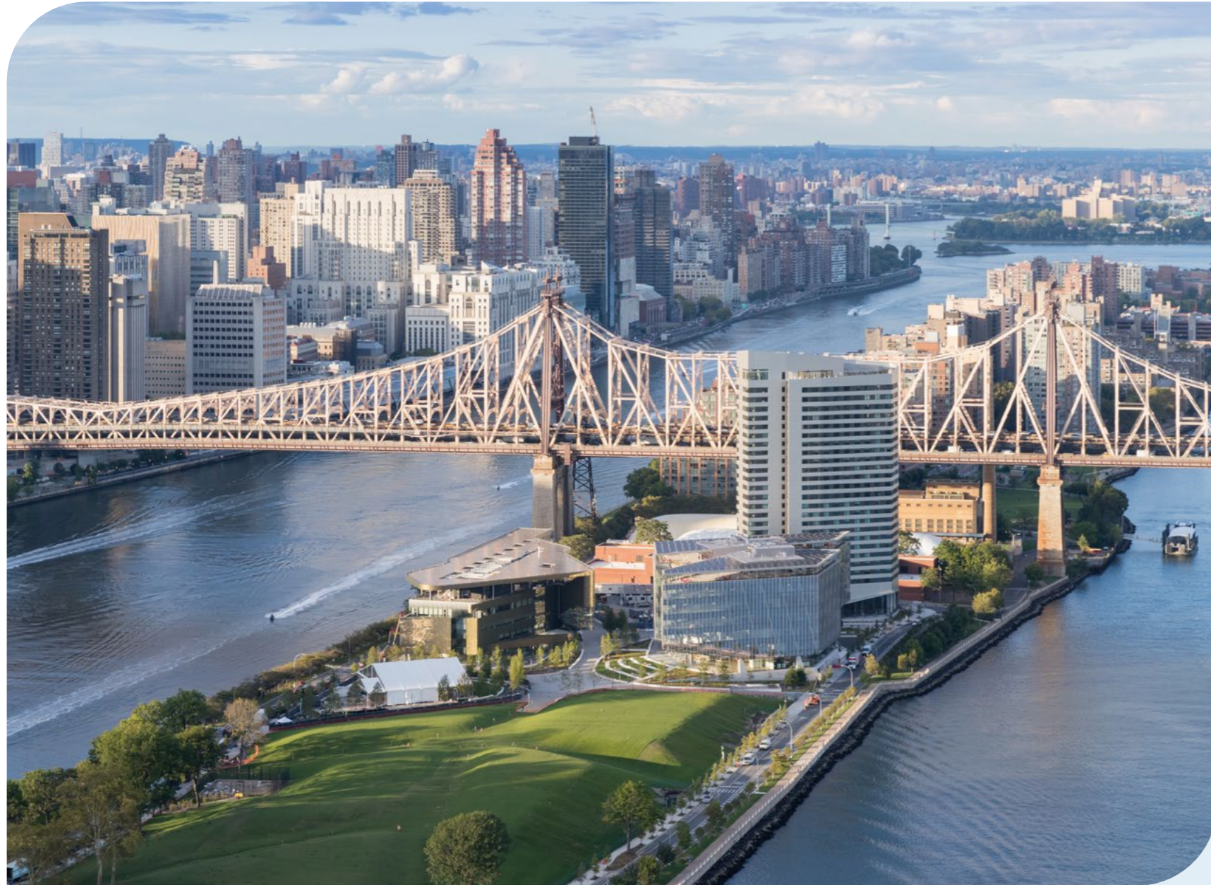
Project of the Year – Public Use, The House at Cornell Tech, Buro Happold
