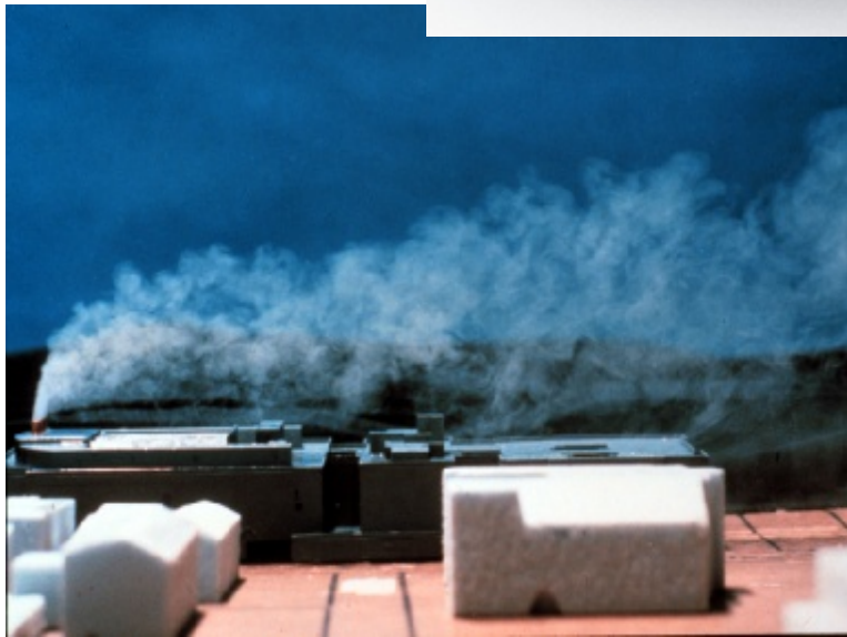
before raising stack height
