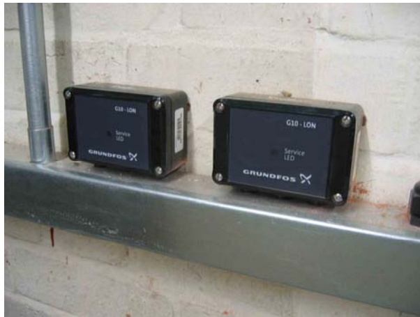
Figure 6: Grundfos pump G10 Lon gateway between manufacturers and LonTalk protocol.
